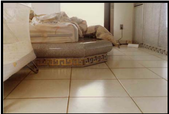
Another platform bed. The goods used on this cost about $200 per sheet. This radius is a 6” radius, and Bruce advised that you can heat the laminate to bend it, you can sand the back as well to make it thinner, or you can order it pre-formed.
