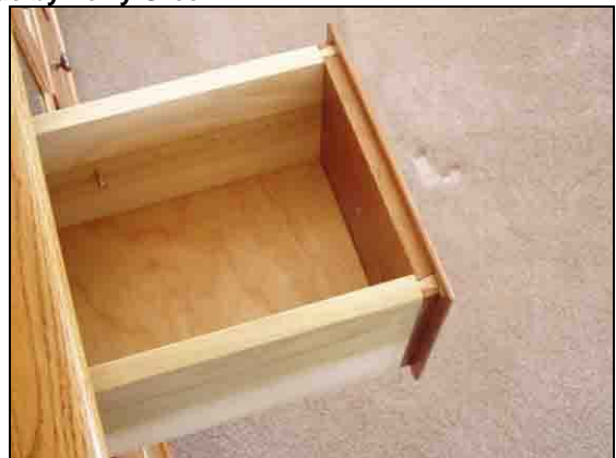
Sliding dovetail drawer sides?
