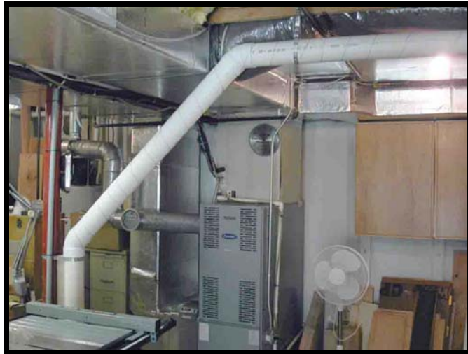
If you are using PVC, two 45's are better than one 90 degree fitting as shown here.
