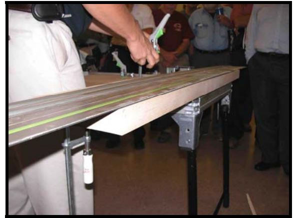
A long guide rail for a long cut in thick stock. It was accomplished easily.
