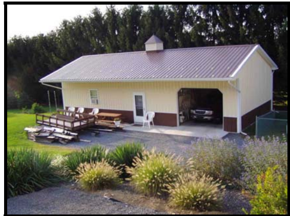
Terry's shop. Built to BE a shop. Building is 24x48, of which 24x32' is workshop. Ceilings are 10' high.
